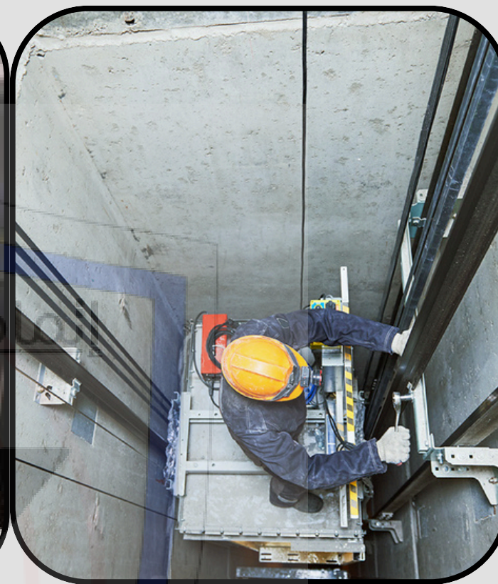
Elevator Maintenance
