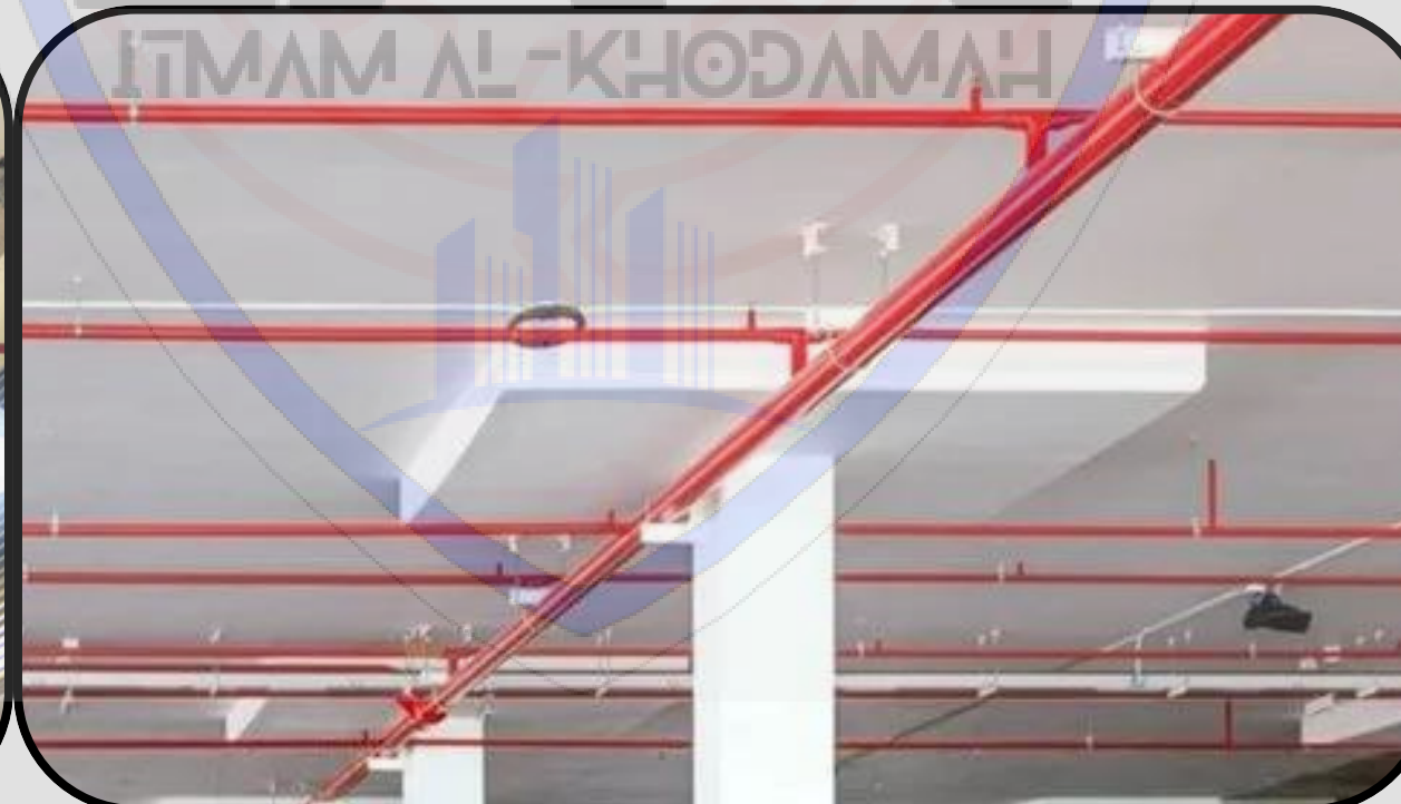
Water Sprinkling System
